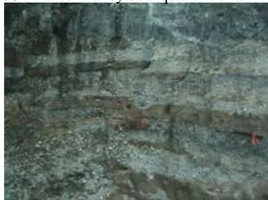
Picture 4-2: Displacement in excavation near Rose Wagner Performing Arts Center
